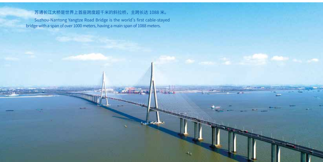
苏通长江大桥 Sutong Yangtze River Bridge
