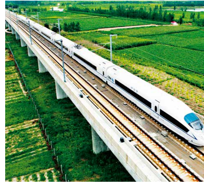
京沪高速铁路 Beijing-Shanghai High-speed Railway
