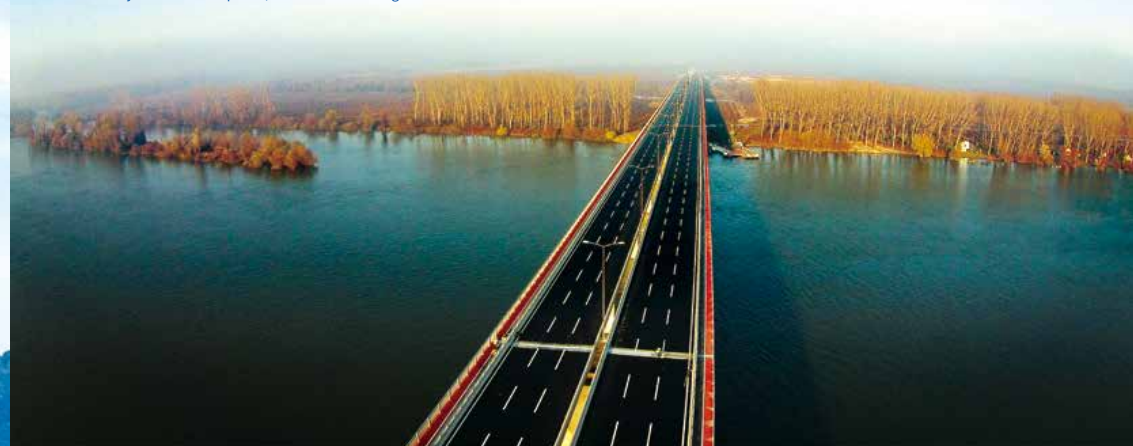
塞尔维亚泽蒙博尔察大桥 Zemun-Borca Bridge in Serbia
