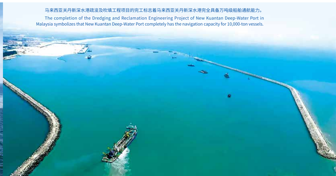
马来西亚关丹新深水港疏浚及吹填工程 Dredging and Reclamation Engineering Project of New Kuantan Deep-Water Port in Malaysia
