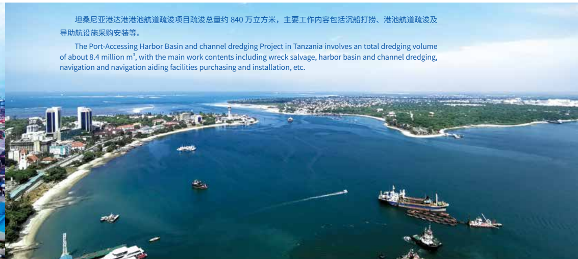
坦桑尼亚港达港港池航道疏浚 Port-Accessing Harbor Basin and Channel Dredging Project in Tanzania
